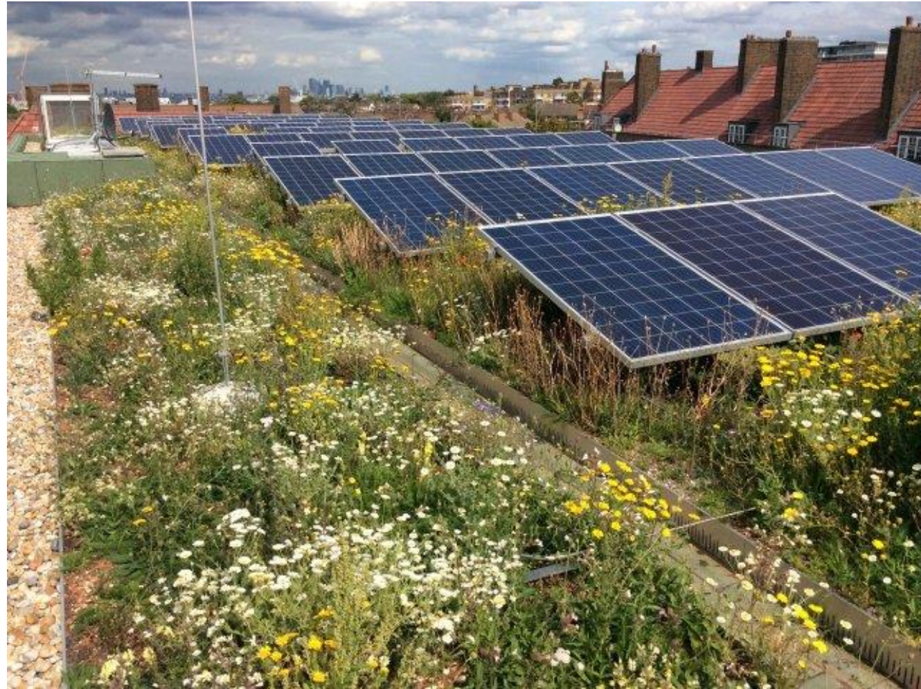
Photo: Clapham Park – Biosolar roof London – Bauder Ltd
