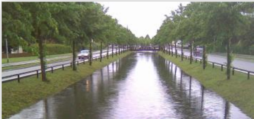
Reopening a canal for storm water management in Växjö , Sweden
